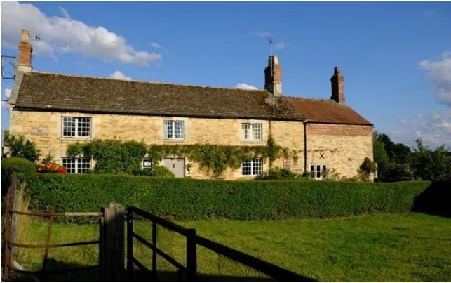
Picture 3 North Luffenham Farm House
